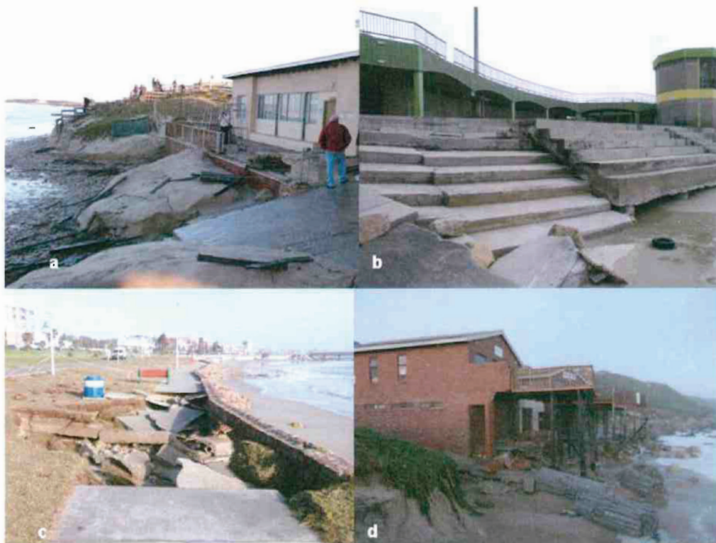
Figure 1-1: Threat to infrastructure placed too close to the sea through erosion at a) Summerstrand lifesavers clubhouse, b) New Brighton Beach facilities and wave attack at c) seawall and walkway east of hobie beach and d) clubhouse facilities at Sardinia Bay.
