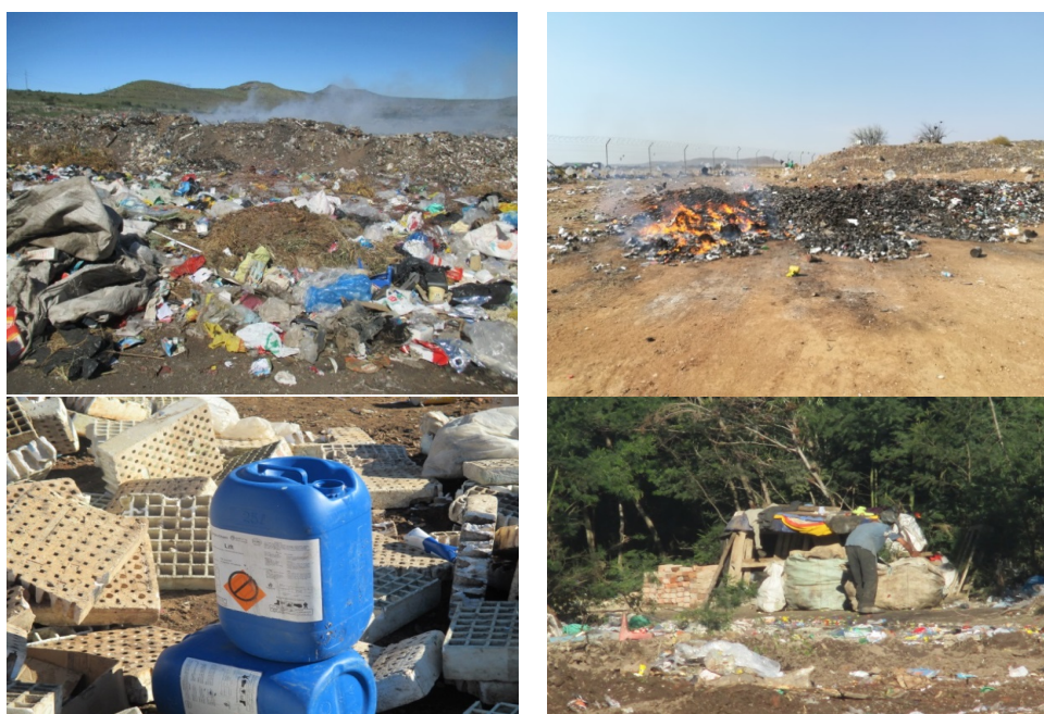
Figure 27. A) Uncovered waste and burning of the landfill site at Cradock landfill site, B) Burning of waste at the Hofmeyr landfill site, C Hazardous waste at the Hankey landfill site, D) Informal reclaimers at the Humansdorp landfill site
